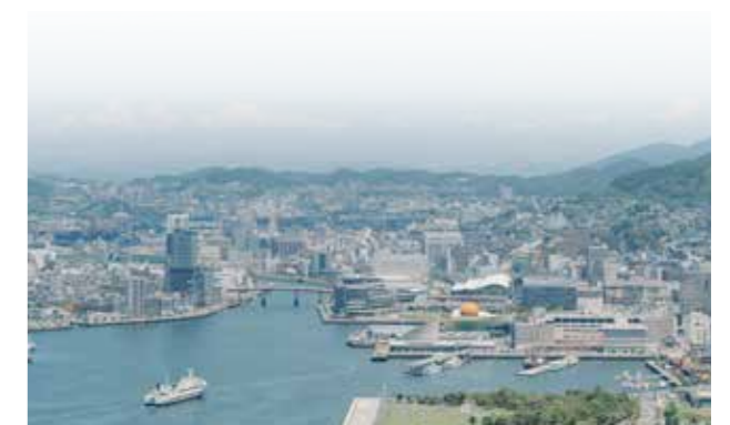
Nagasaki Prefecture Disaster Prevention Administrative Radio Communication System
